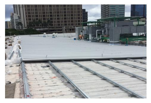
standing seam tabs. The clip design will accommodate expansion and contraction movement in roofs up to 500 feet wide.
